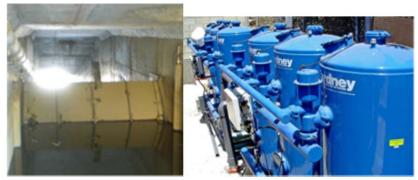
Marie Canyon Low-Flow Diversion – Flat Gate Diverting flow to treatment unit for bacteria
